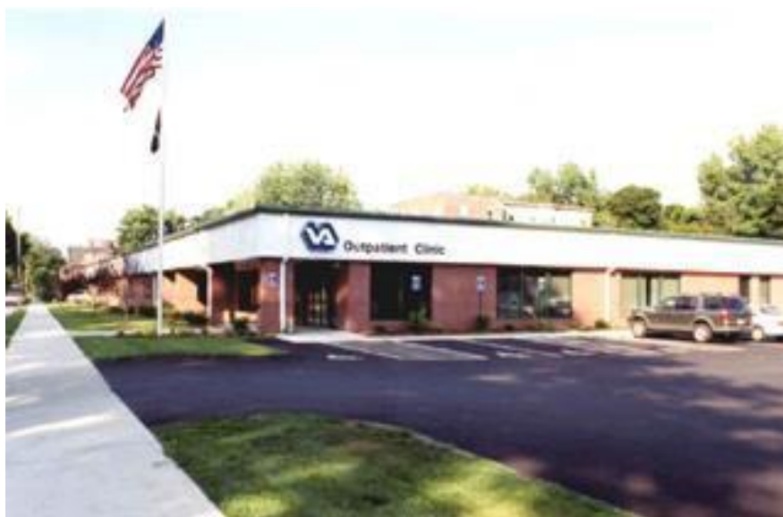
Figure 3: Photograph of the exterior of the Springfield VA Clinic - a single story building with adjacent parking lot and sidewalk
