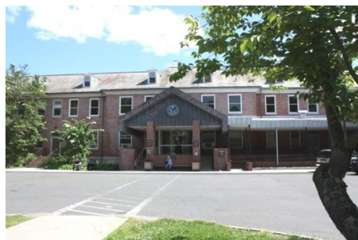
Figure 2: Exterior photograph of Building 1-Liberty, VA CWM-Leeds Campus
